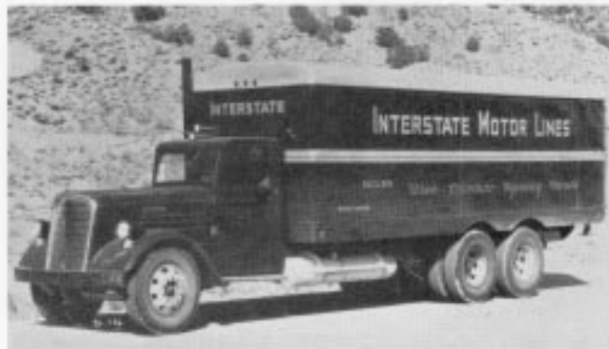
1936 INTERSTATE MOTOR LINES VAN Chain Drive — Also Pulled Full Trailer
